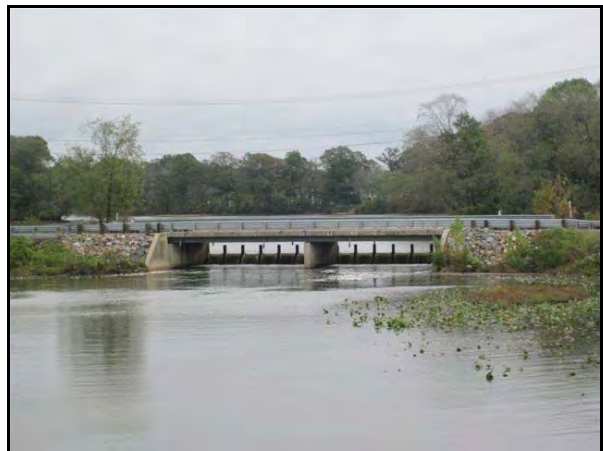
Williams Pond Dam, Seaford, Delaware, Sussex County. By F. Matthew Blaine.
