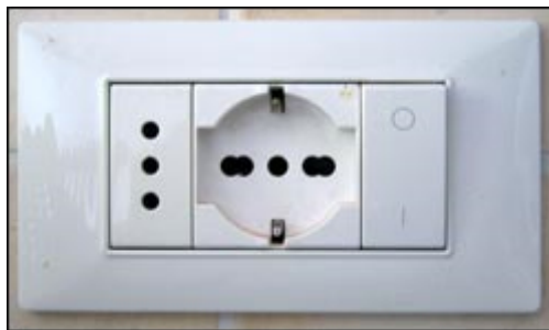
Italian power outlet with a typical power socket, a Schuko Grounded socket for large appliances, and a power switch. An adapter plug will fit into the two outer holes of either socket.
